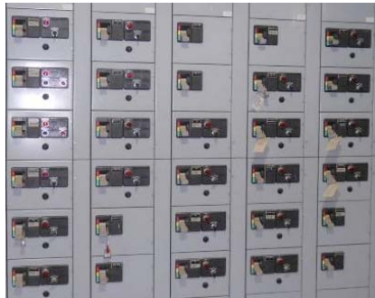
Low Voltage Motor Control Center
