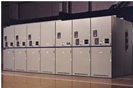
Medium Voltage Switchgear
