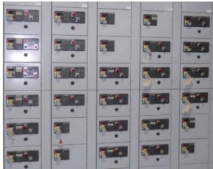
Low Voltage Motor Control Center
