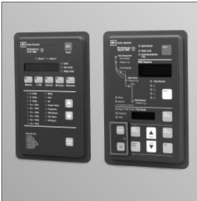
Figure 1-3 A Digitrip 3000 Protective Relay (right) Installed on a Metal Assembly Panel with a DP-4000 (left)
